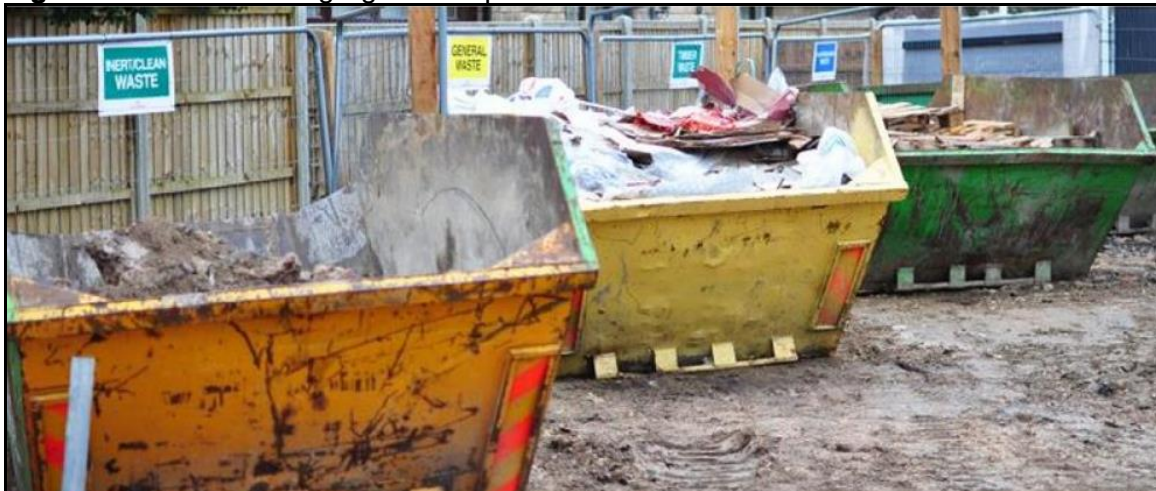
Figure 2 Waste segregation skips
